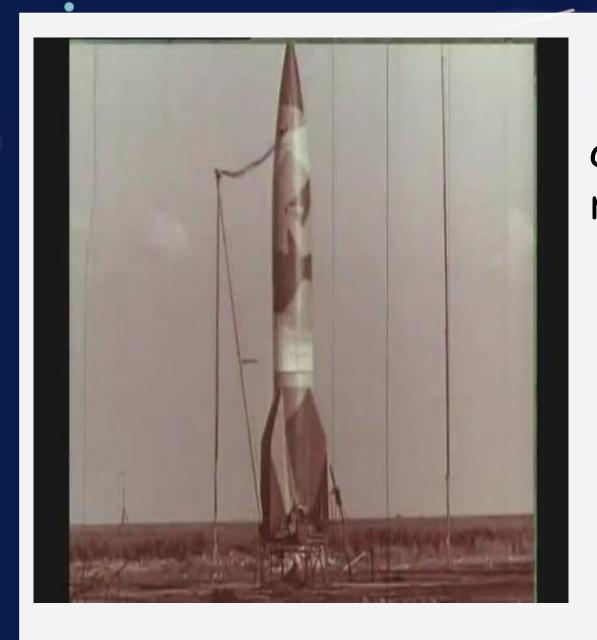
The only problem with using gunpowder was that it wasn't quite powerful enough to push rockets out of Earth's gravity field. During the Second World War, Nazi scientists started to experiment with different fuels to build bigger and more powerful rockets. They designed the V2 rocket to be launched at cities like London.
